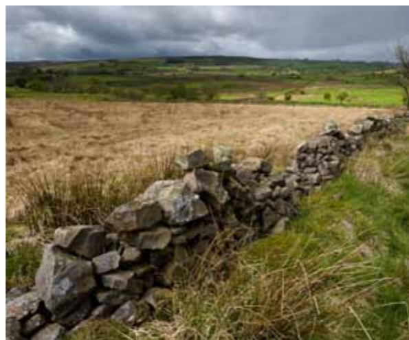
Crumbling walls © PDNPA
