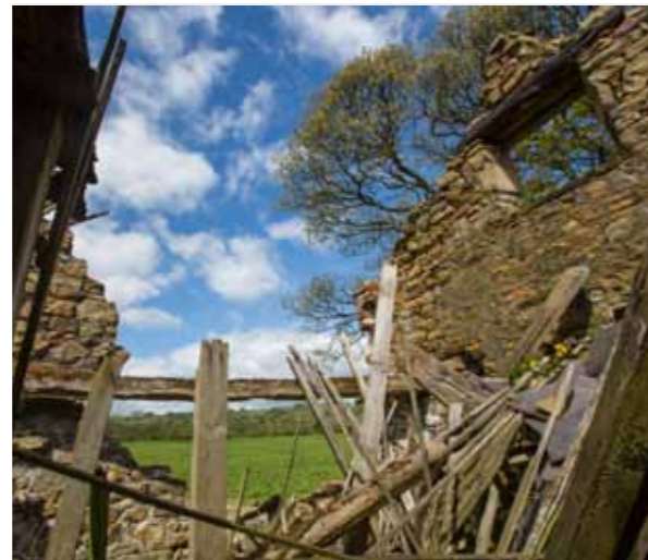
Collapsed field barn © PDNPA
