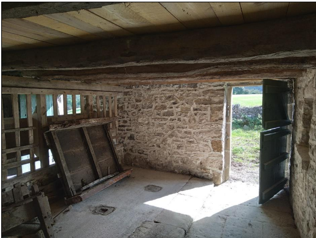
Fig. 23 the sledge in the restored barn
