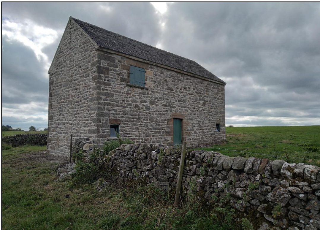
Fig. 14 Hobcroft barn after restoration work
